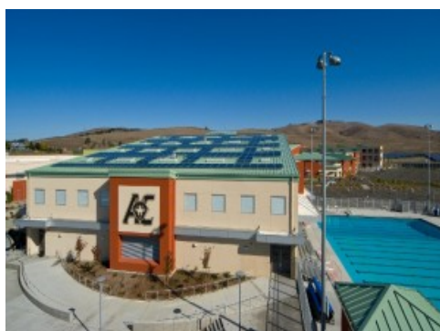
At American Canyon High School, 4,000 solar panels on the roof and on the ground generate 80 percent of the needed electricity. (Photo by Quattrocchi Kwok Architects.)
