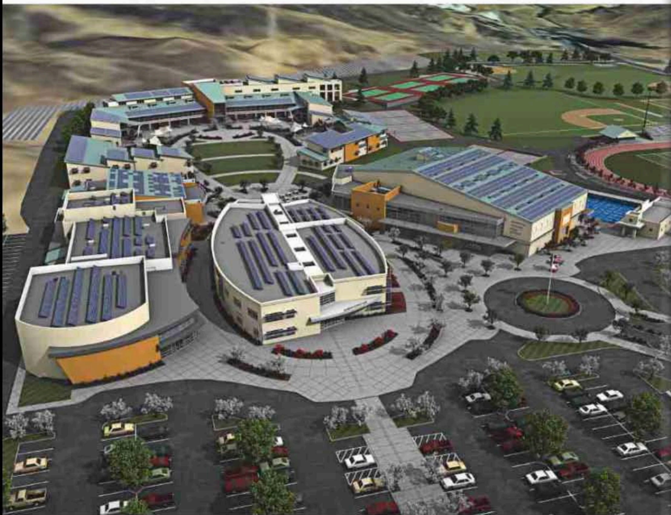
The buildings and pathways of American Canyon High School were designed and oriented to take advantage of sunlight and wind ventilation. The "infinity" pathway that goes past all of the school's buildings also gives students and faculty a view of the greater Bay Area past its entrance.
